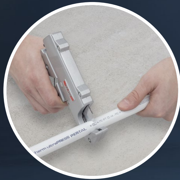
01 | Cutting the pipe with pistol or roller shears.
